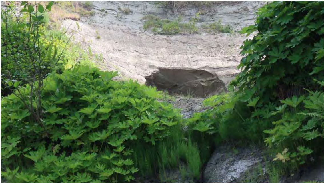
Site of recent sand blowout from perched groundwater just above the silt clay layer at bluff northwest of the mine.
